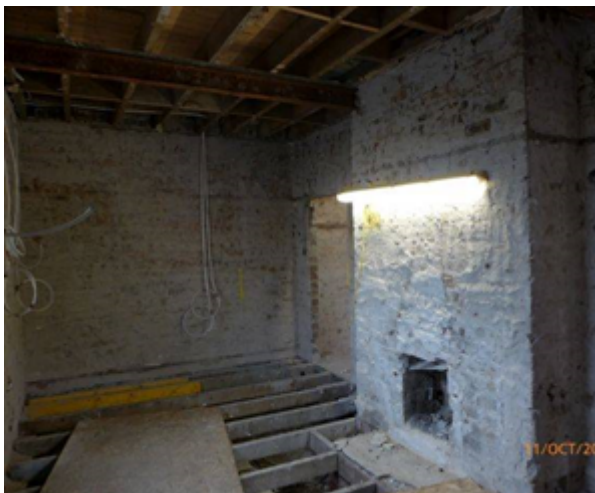
Ground Floor: General View.
