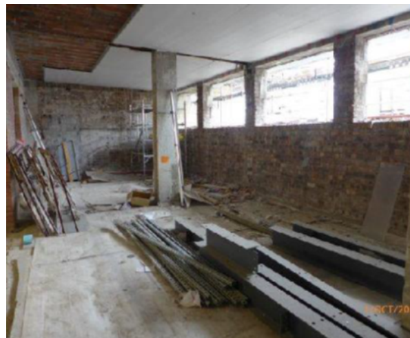
Exhibition Space (East Elevation – Argyle St.): Removal of existing external windows and installation of new Crittall windows.
